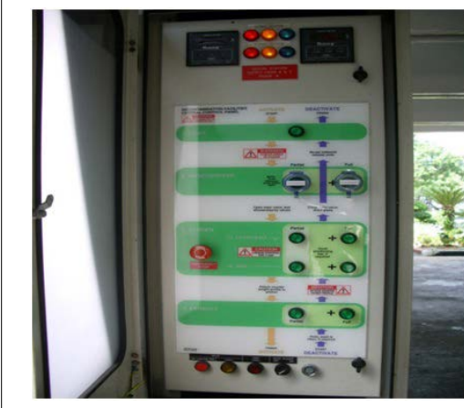
Figure 4. Control panel for activation of Hospital Decontamination Station with Options for Partial or Full Deployment
