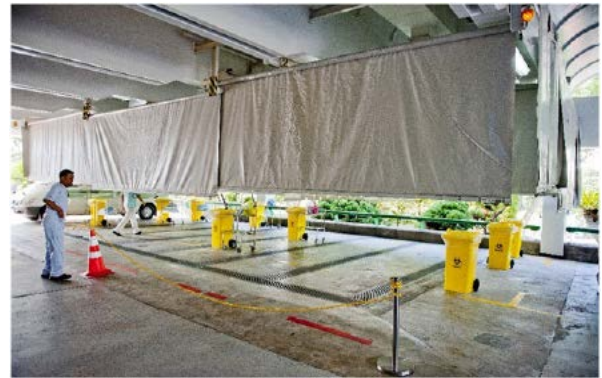
Figure 1B. Deployment of Hospital Decontamination Station (HDS) Shower Curtains
